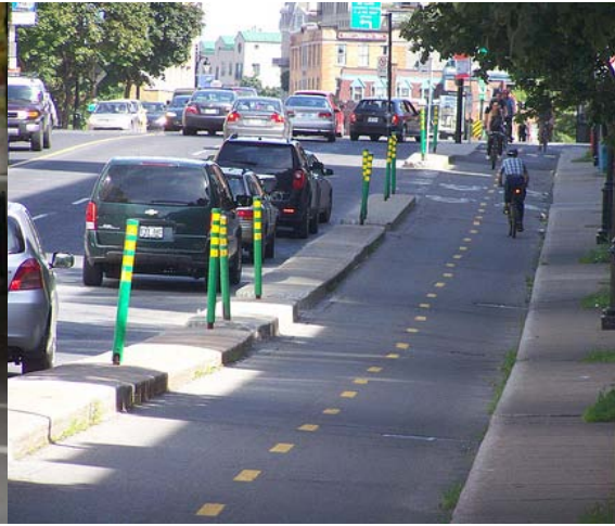
Two-way Street Level Cycle Track, Separated by a Median in Montreal, PQ 11
