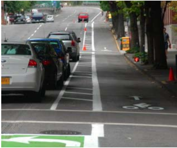
One-way Street Level Cycle Track, Adjacent to Parking in Portland, OR 10
